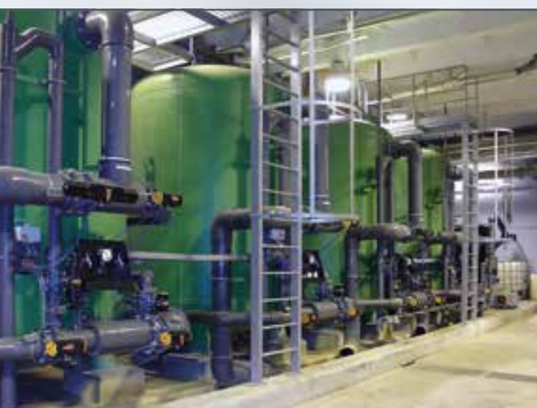
Continuous-flow adsorber in a water treatment plant
