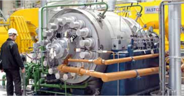
A centrifugal pump at a power plant
