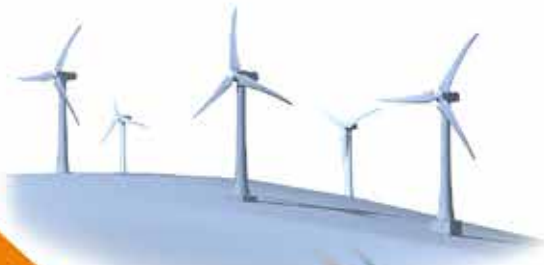
Wind power plant
